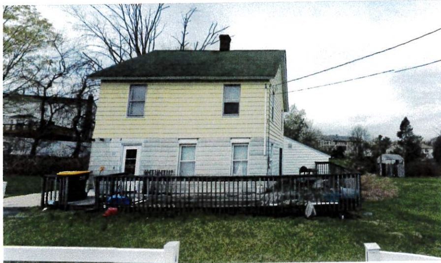
EXISTING FRONT PHOTOGRAPH
