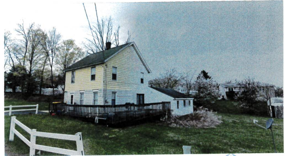
EXISTING FRONT RIGHT CORNER PHOTOGRAPH
