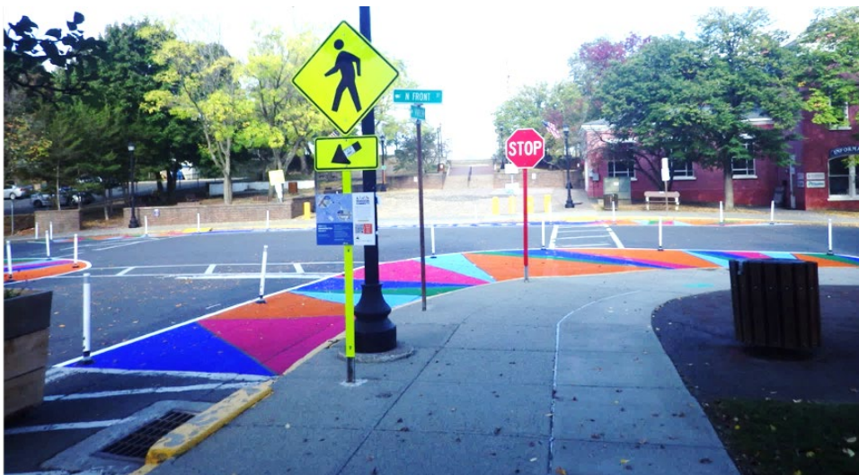
Painted bump-outs with flexible bollards installed as part of Creighton Manning's streetscape improvements in Hudson
