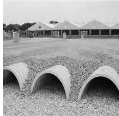
Small dozers and skid loaders may be used to finish grading stone backfill in accordance with ground pressure limits in Table 2. They must push material parallel to rows only. Never push perpendicular to rows. StormTech recommends that the contractor inspect chambers before placing final backfill. Any chambers damaged by construction shall be removed & replaced.
