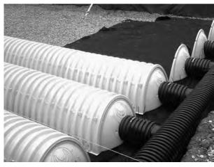
Align the first chamber and end cap of each row with inlet pipes. Contractor may choose to postpone stone placement around end chambers and leave ends of rows open for easy inspection of chambers during the backfill process.
