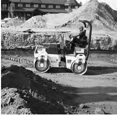
Install non-woven geotextile over stone. Geotextile must overlap 24" (600 mm) min. where edges meet. Compact each lift of backfill as specified in the site design engineer's drawings. Roller travel parallel with rows.
