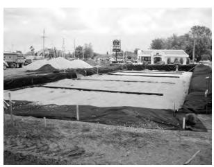
Place clean, crushed, angular stone foundation 6" (150 mm) min. Install underdrains if required. Compact to achieve a flat surface.
