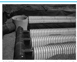
24" (600 mm) inlets are the maximum size that can fit into a SC-740/DC-780 end cap and must be prefabricated with a 24" (600 mm) pipe stub. SC-310 chambers with a 12" (300 mm) inlet pipe must use a prefabricated end cap with a 12" (300 mm) pipe stub.
