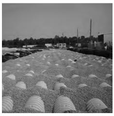
Continue evenly backfilling between rows and around perimeter until embedment stone reaches tops of chambers. Perimeter stone must extend horizontally to the excavation wall for both straight or sloped sidewalls. Only after chambers have been backfilled to top of chamber and with a minimum 6" (150 mm) of cover stone on top of chambers can small dozers be used over the chambers for backfilling remaining cover stone.
