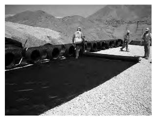
Install manifolds and lay out woven scour geotextile at inlet rows [min. 12.5 ft (3.8 m)] at each inlet end cap. Place a continuous piece (no seams, double layer) along entire length of Isolator® Row(s).
