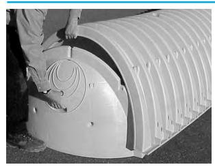
Lift the end of the chamber a few inches off the ground. With the curved face of the end cap facing outward, place the end cap into the chamber's end corrugation.
