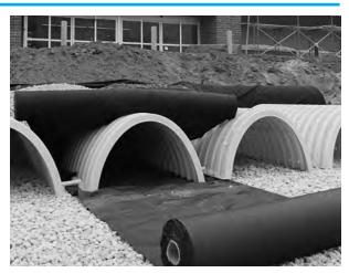
Drape a strip of ADS non-woven geotextile over the row of chambers (not required over DC-780). This is the same type of non-woven geotextile used as a separation layer around the angular stone of the StormTech system.
