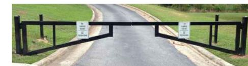
Simple steel hinge gate for emergency access drive. To be fitted with a mechanism on the hinges that will open with the sound of an emergency siren.
