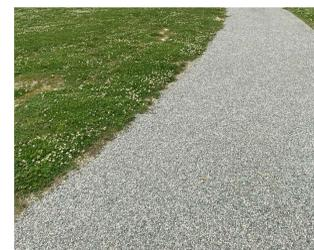
Gravel is pressed into asphalt pavement to create Chipseal. Reduces slipping and glare from wet surfaces, prolongs the life of asphalt.
