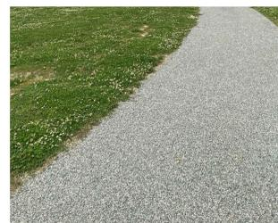
Gravel is pressed into asphalt pavement to create Chipseal. Reduces slipping and glare from wet surfaces, prolongs the life of asphalt.
