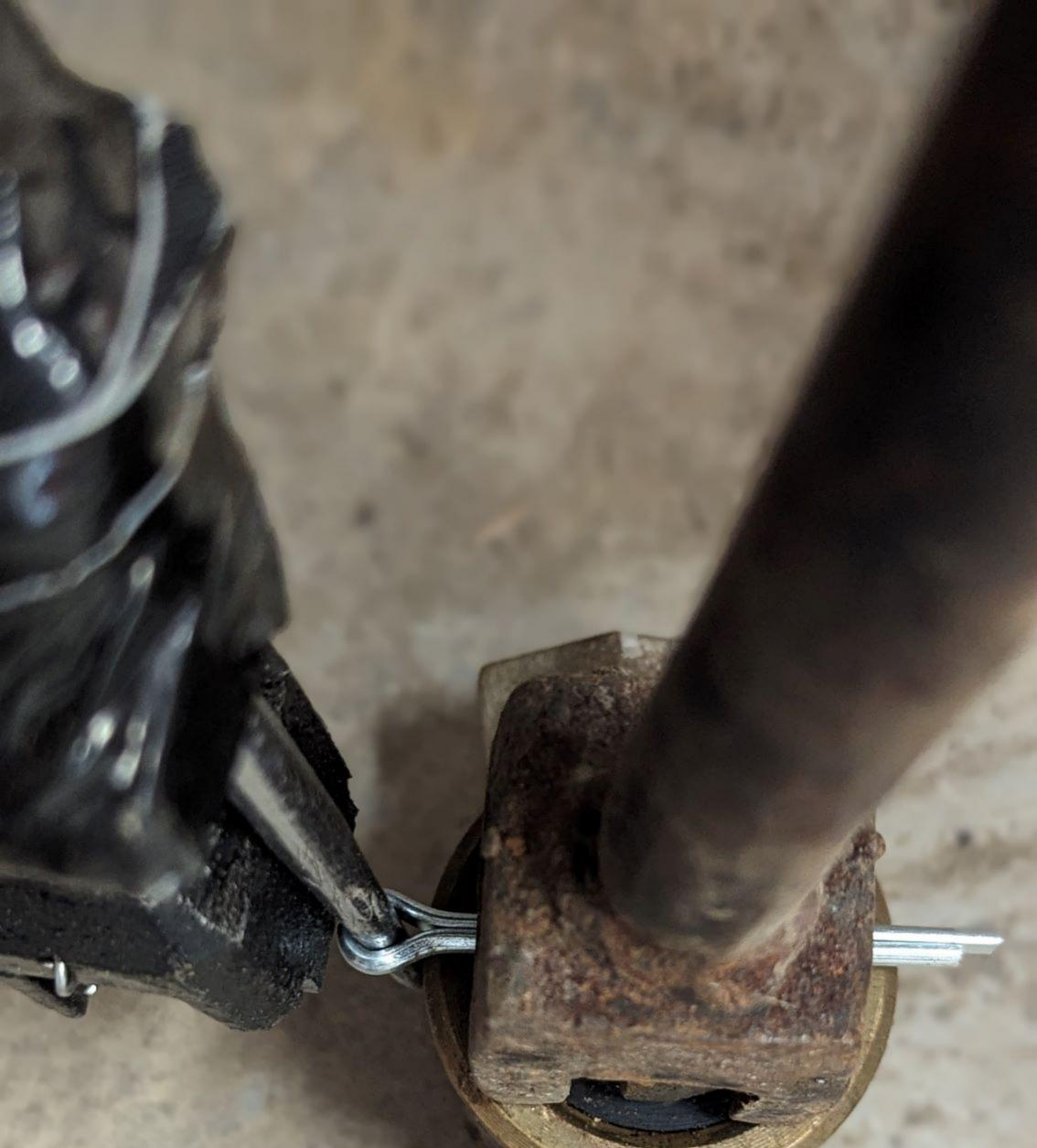
Sliding the new pin through the valve and rod
