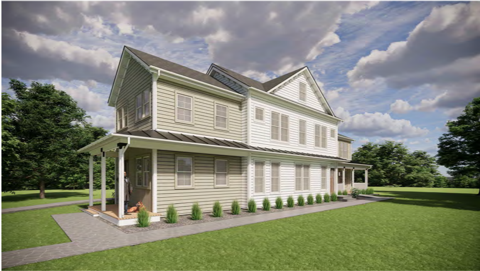
FRONT LEFT CORNER
