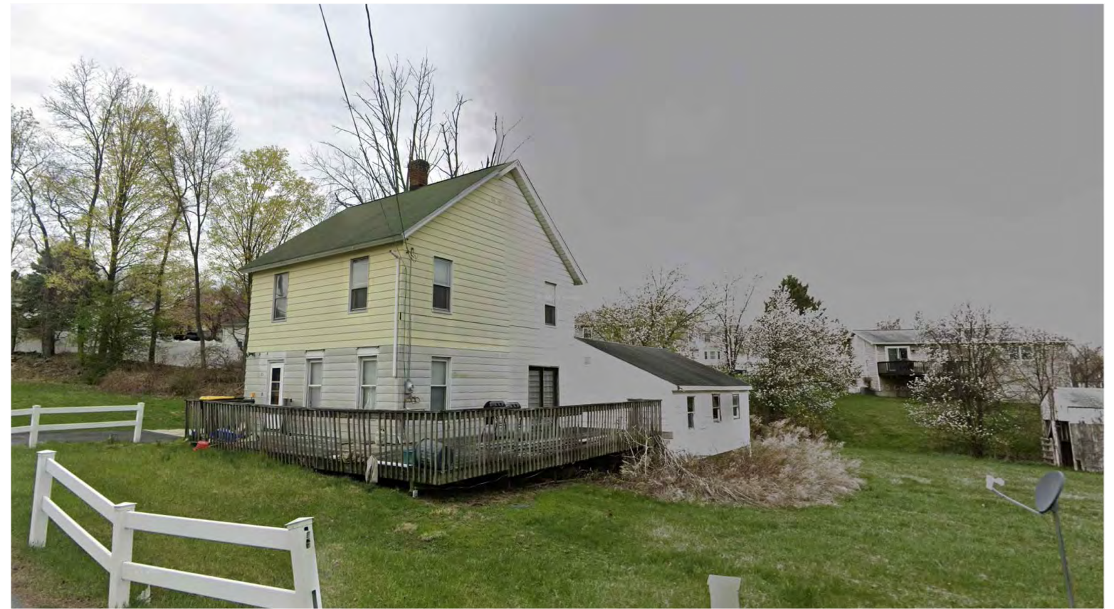
EXISTING FRONT RIGHT CORNER PHOTOGRAPH
