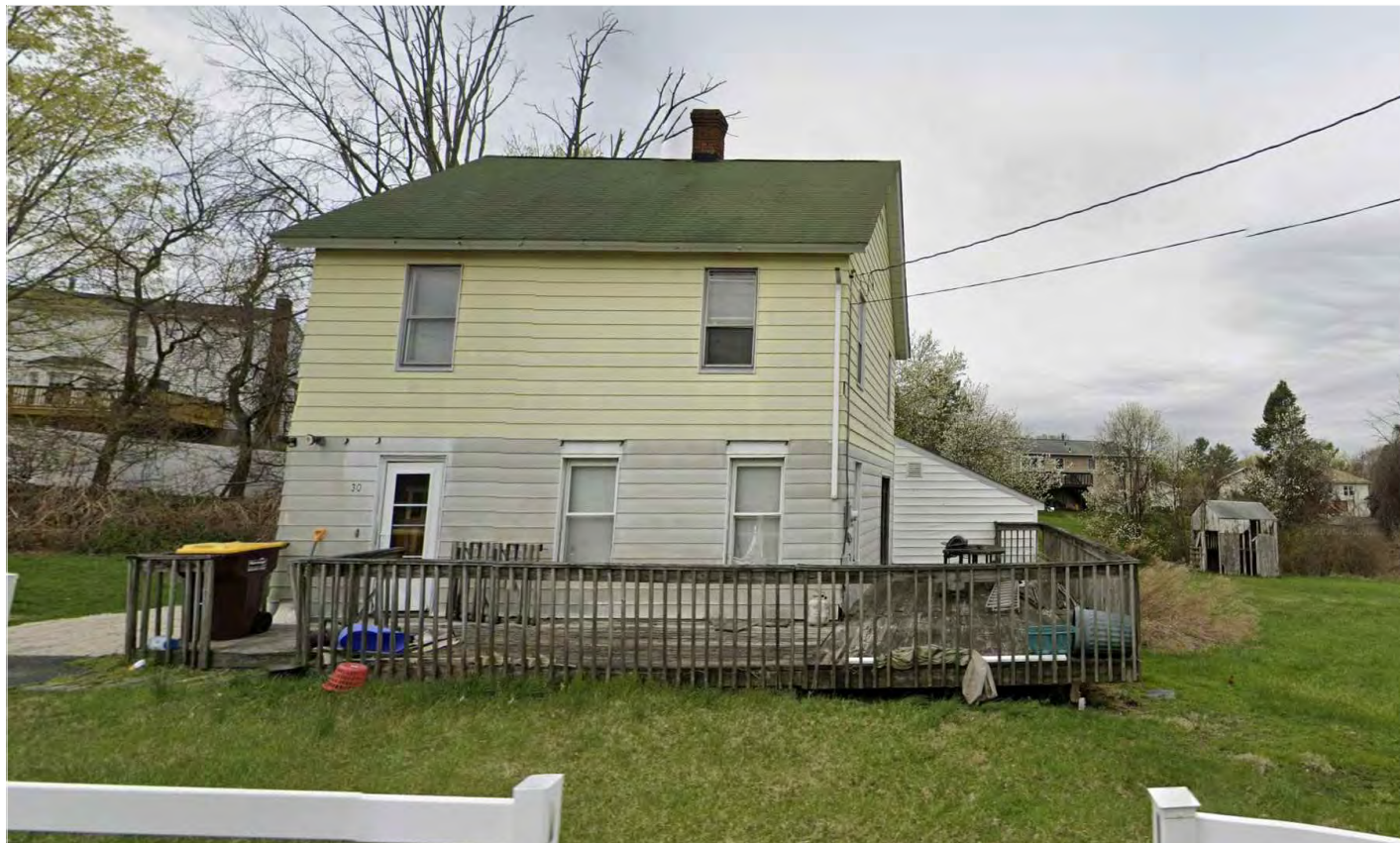
EXISTING FRONT PHOTOGRAPH
