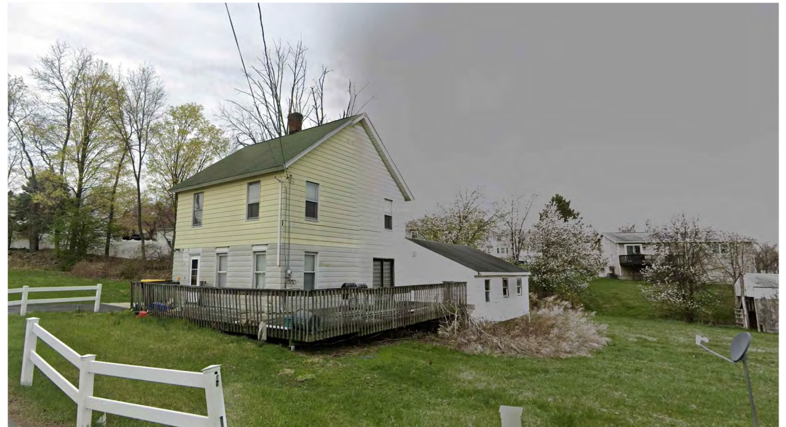
EXISTING FRONT RIGHT CORNER PHOTOGRAPH
