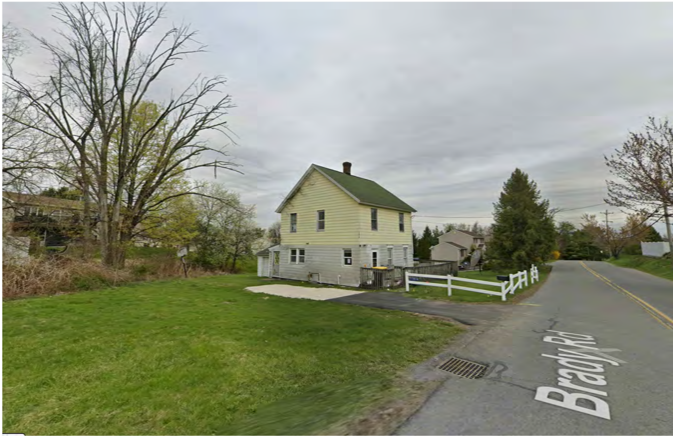
EXISTING STREET VIEW
